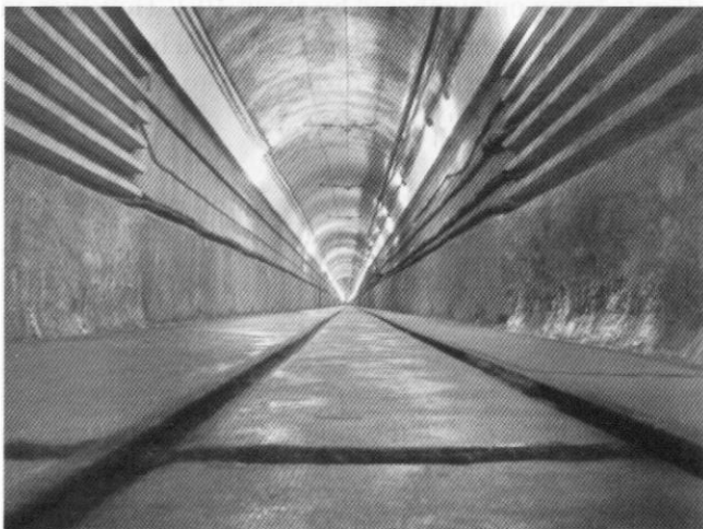
Main corridor at Fort Schoenenbourg
